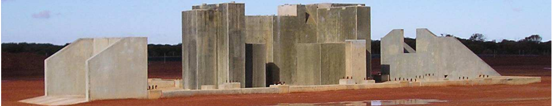
Mount Weld Concentration Plant site – Ball Mill foundations
